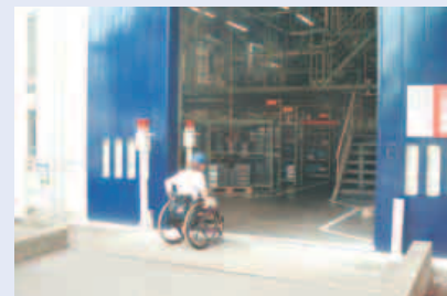
The entrance of the Oizumi Plant, equipped with a wheelchair ramp and an automatic door
