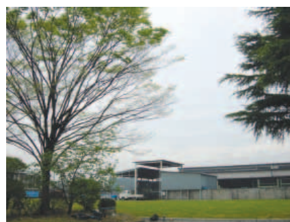
The vacant lot of the incinerator in the Yajima Plant in the Gunma Manufacturing Division is now green space.
