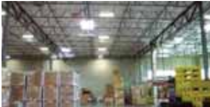
(Picture 9) SOA's Lamp replacement project
