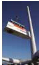
⑤The nacelle being lifted to the tower
