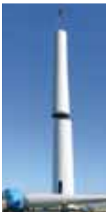
③The 62-m-high tower being constructed
