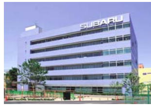
Omiya Business Site
