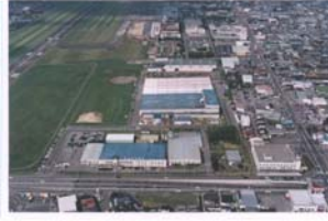
South No.2 Plant
