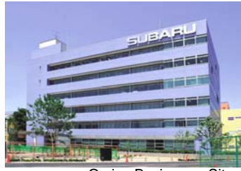
Omiya Business Site
