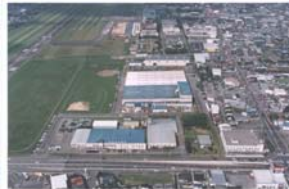
South No.2 Plant
