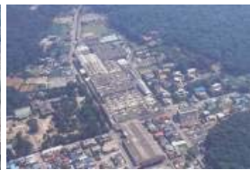
Ota North Plant
