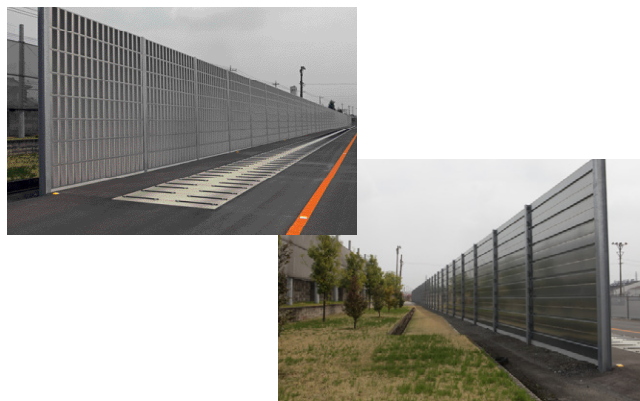
Soundproof fence erected giving due consideration to green space
