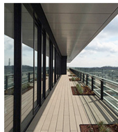
Solar radiation shielding due to the effect of the balcony eaves
