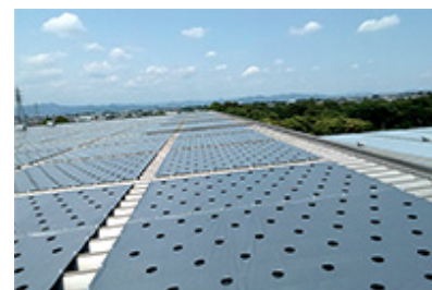
Insulation sheets attached to a plant roof
