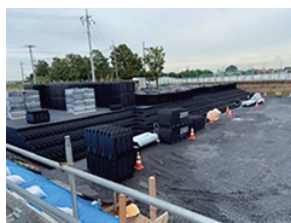
Construction of the storm water detention tank
