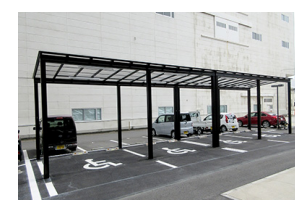
Parking for wheelchair users (West Main Building, Gunma Plant)
