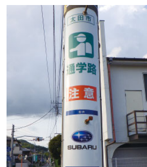
Installing Signs on Utility Poles
